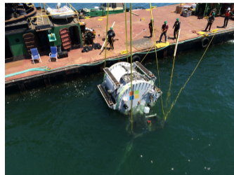
Microsoft's project Natick: immersed datacenter
